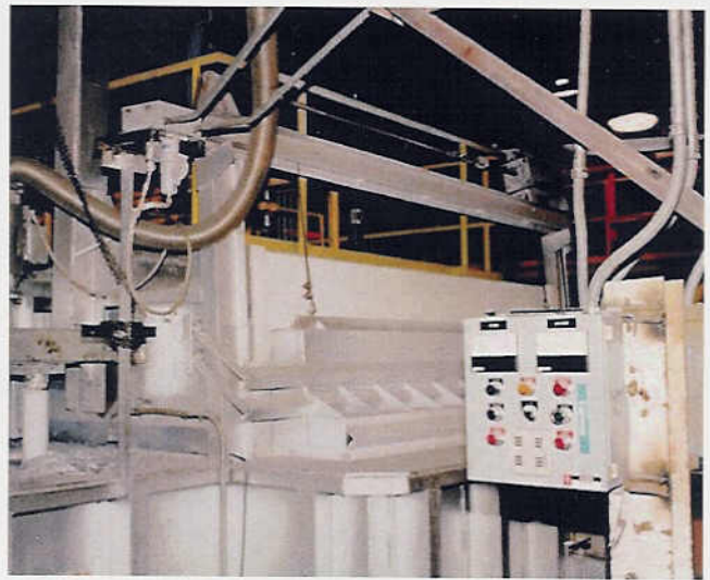
Figure 5: Circulation well and pump.
