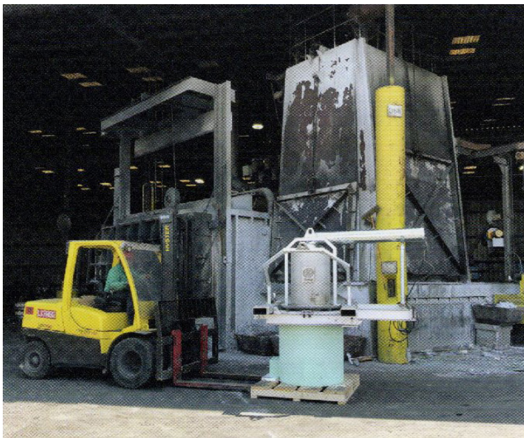
Figure 1. The side-well furnace at the Fontana operation was outfitted with a new MagPump (seen in front), which replaced the existing mechanical pump.
